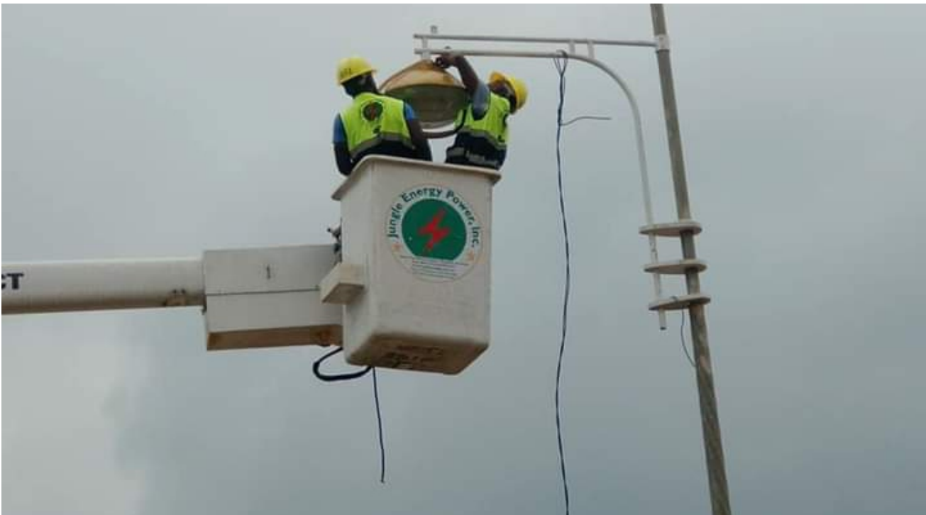
JEP Technicians install street lights
