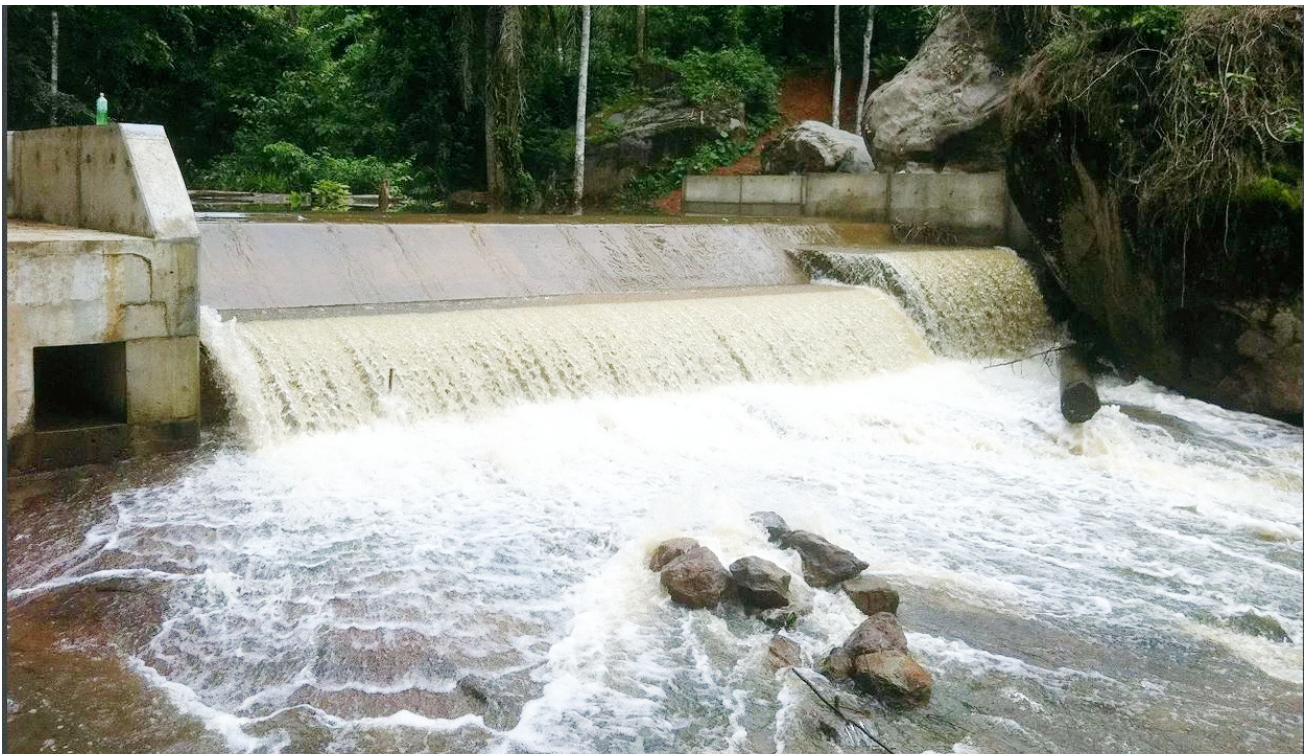
Yandohun Micro Hydro Power Plant
