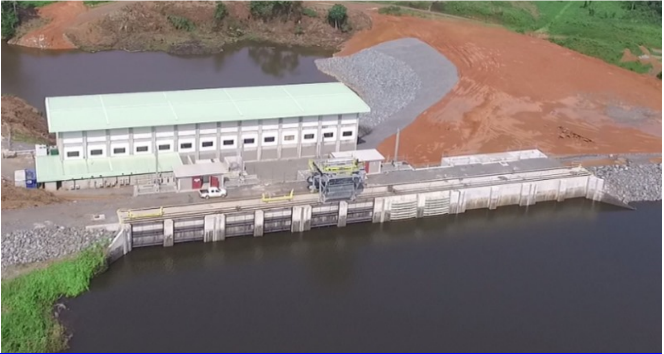
Mount Coffee Hydropower Plant
